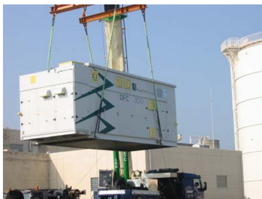
熔融炭酸塩形 FuelCell Energy, DFC® 300A 250 kW MCFC
